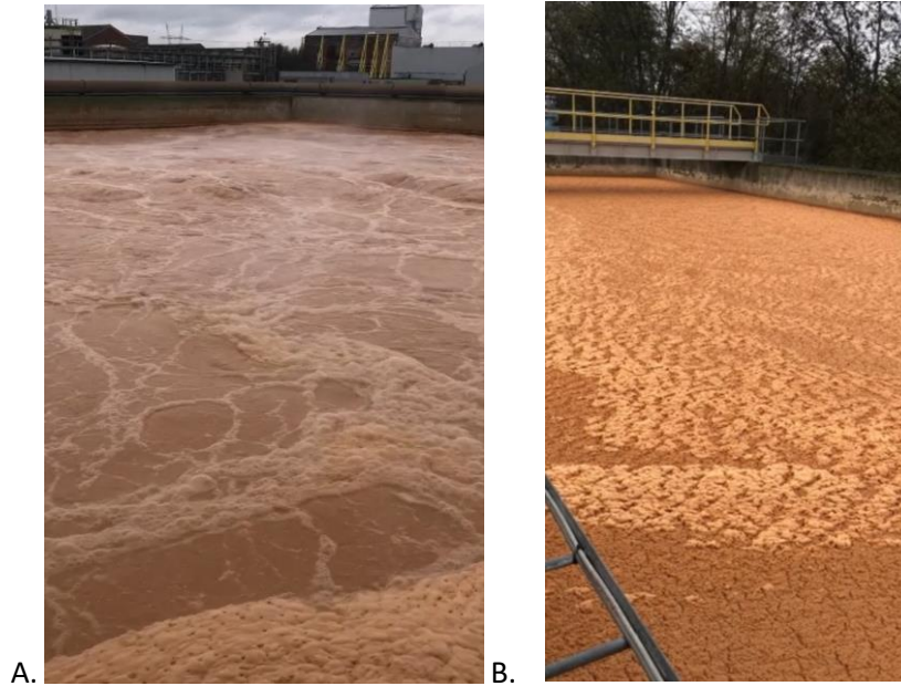
Figure: The basin of the PB Leiner wastewater treatment plant in A) nitrification modus and B) denitrification modus.
