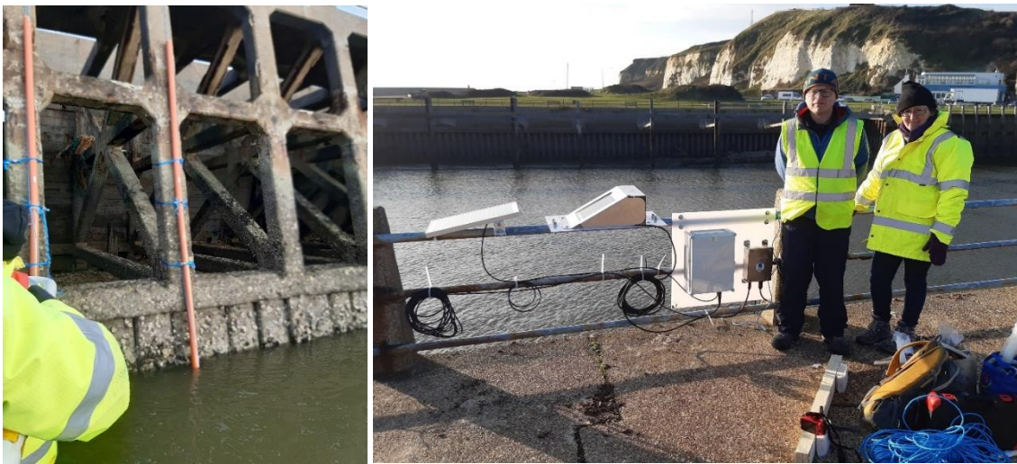
Figure NH8: Photographs of the final installation, Newhaven Port.
