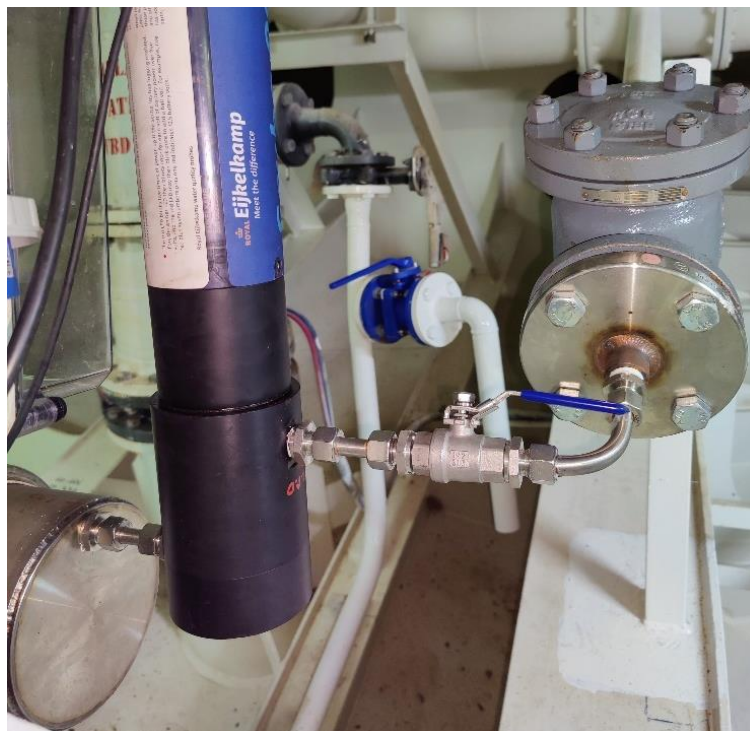
Figure 31: Flow cell of the Scuba sensor (left), reducer and check valve (right).
