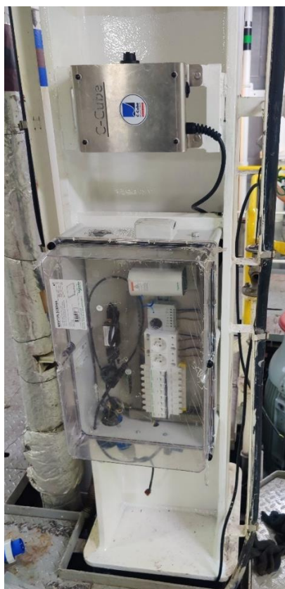
Figure 19: Mounting of the electrical cabinet and C-Cube logger box.
