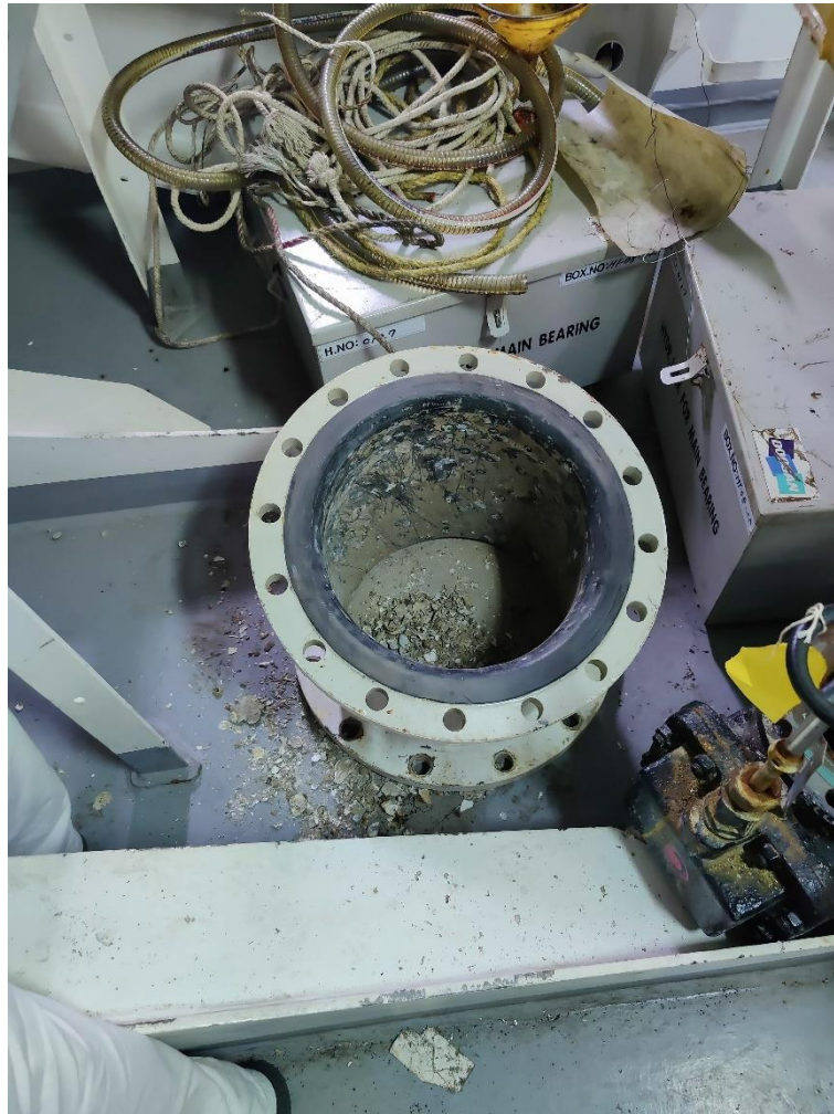
Figure 21: Polyethylene lining in a piece of pipe
