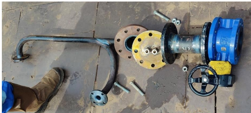
Figure 16. The various parts of the modified vent pipe.
