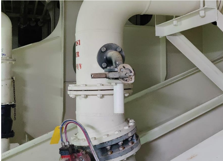
Figure 26: The original sample point on ballast water overboard line
