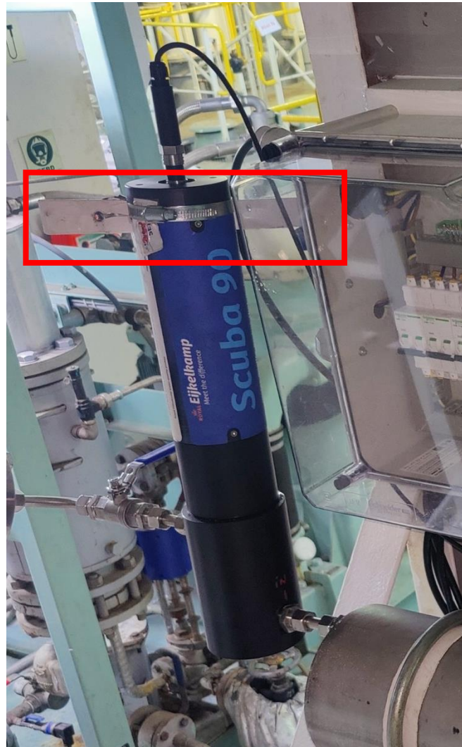
Figure 33: Scuba sensor mounting method.
