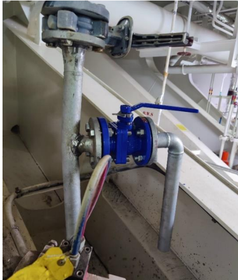
Figure 27: The T-piece attached to the original valve (top) and the new sampling point (right).
