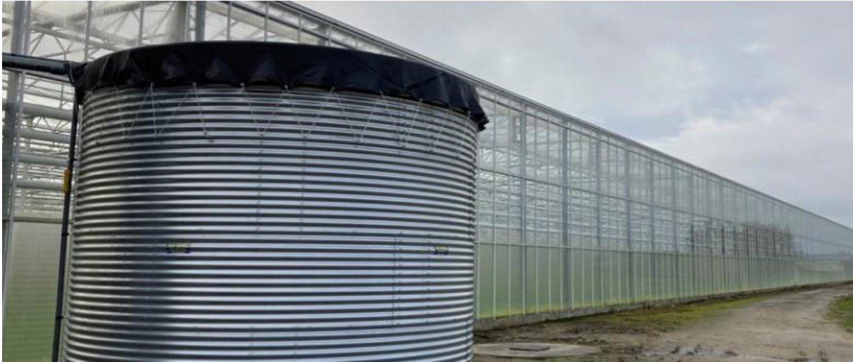
Figure: the MBBR installation next to the greenhouse, in Putte (Flanders).
